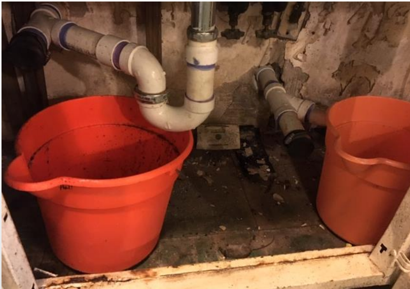
Leaking Pipes
