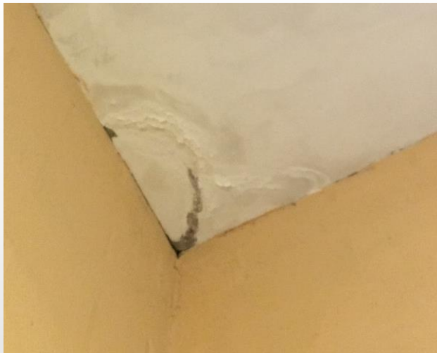
Water Damage
