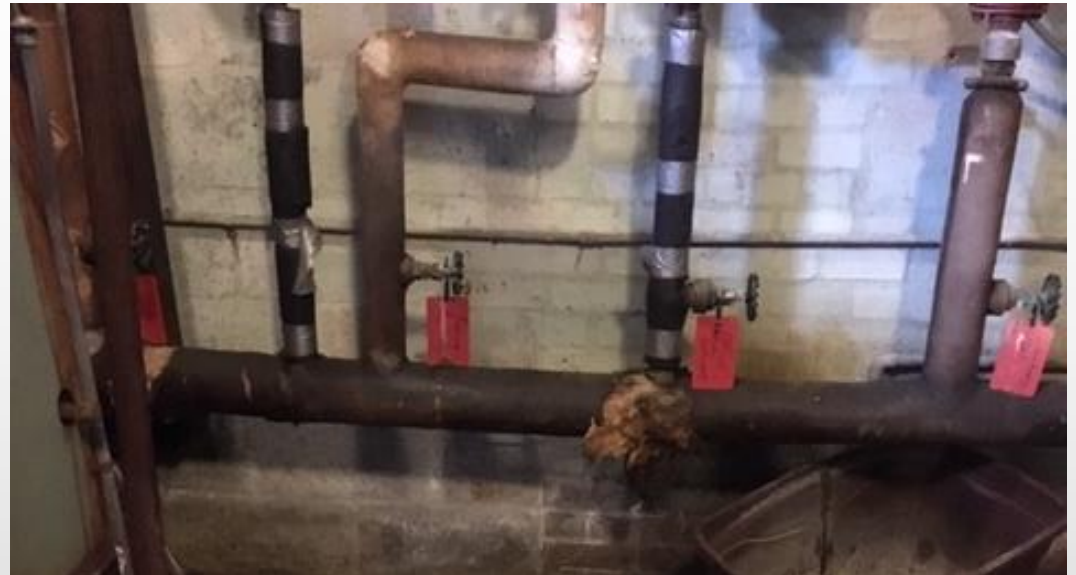
Leaking Pipes
